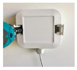
Ensure that the cable gland is fully tightened. Open the hatches on the front of the casing and drill two screws into the wall.
